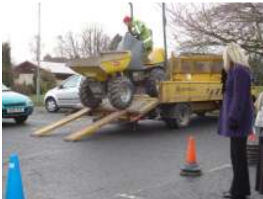
The dumper truck rolls into place.
